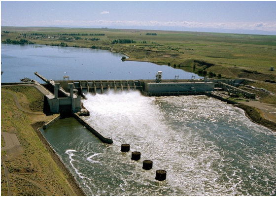
Figure 1: Ice Harbor Dam on the Snake River near Burbank, WA from U.S. Army Corps of Engineers. Ice Harbor Lock and Dam , nwd.usace.army.mil/Media/Images/igphoto/2000790239/
