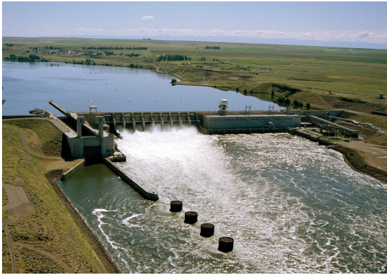
Figure 1: Ice Harbor Dam on the Snake River near Burbank, WA from U.S. Army Corps of Engineers. Ice Harbor Lock and Dam , nwd.usace.army.mil/Media/Images/igphoto/2000790239/
